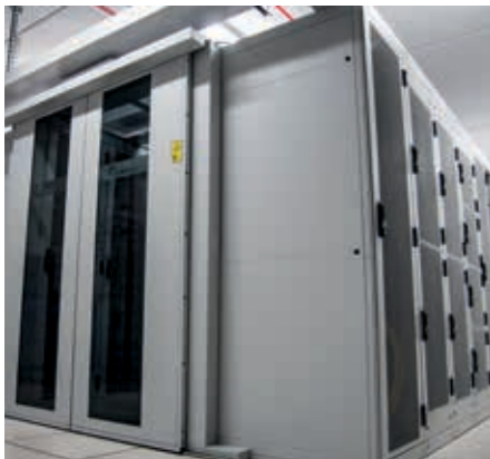
The Minkels Cold Corridor ensures and optimises data centre cooling while taking the heat generated by the servers into account.
