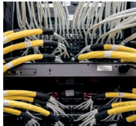
LCS 2 cable solutions by Legrand, both optical fibre and copper cables (Cat. 6A).
