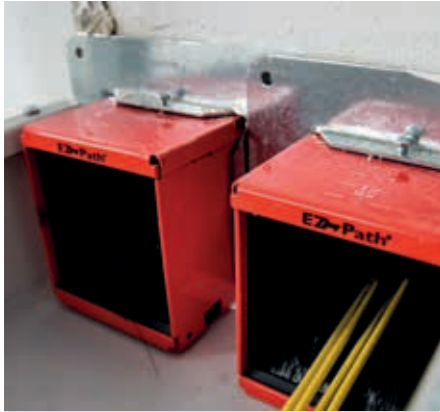
The EZ-Path® firewall module by LCM (Legrand Cable Management) enables organised cable installation through walls, without risk of flashover.
