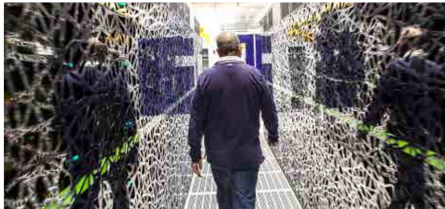
Jim Jansen, Operativer Engineer Datacenter bei Vancis
