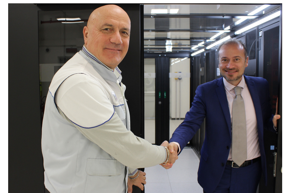
Poalo De Nardis (IT manager) and Floriano Monteduro (Legrand Data Center Solutions)
