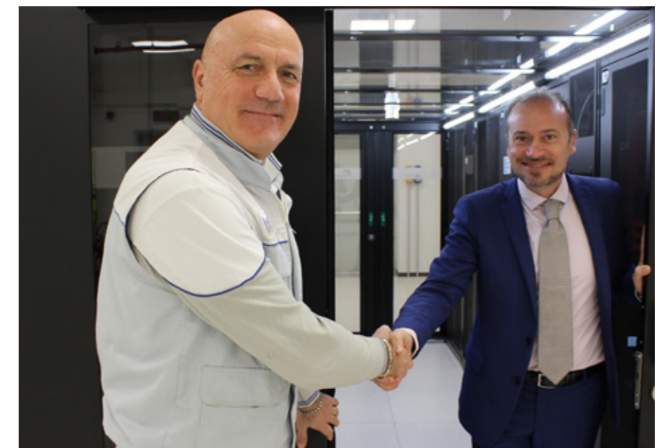
Poalo De Nardis (IT manager) and Floriano Monteduro (Legrand Data Center Solutions)
